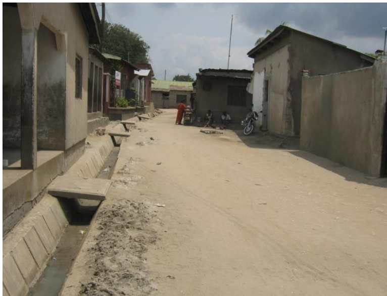
Figure 5: Housing extension obstructing MN1-2 road at Mnyamani settlement
